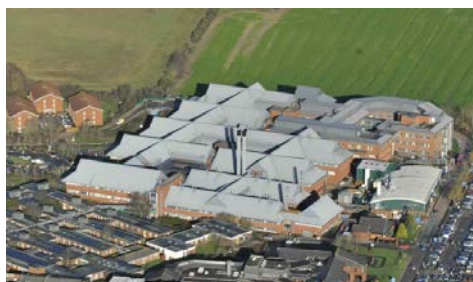
SDH North viewed from the South
