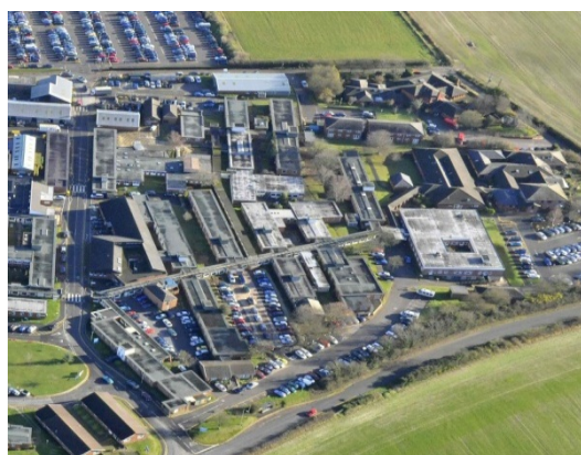
SDH South Viewed from the West
